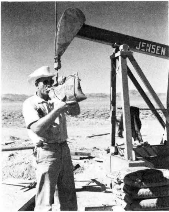
CLEM ROLLINS was range support section supervisor during the early days. Later he joined REECO, the company that constructed and still provides support operations at TTR. The well is the first one at the Range; it went dry during an earthquake in the early 60s.
